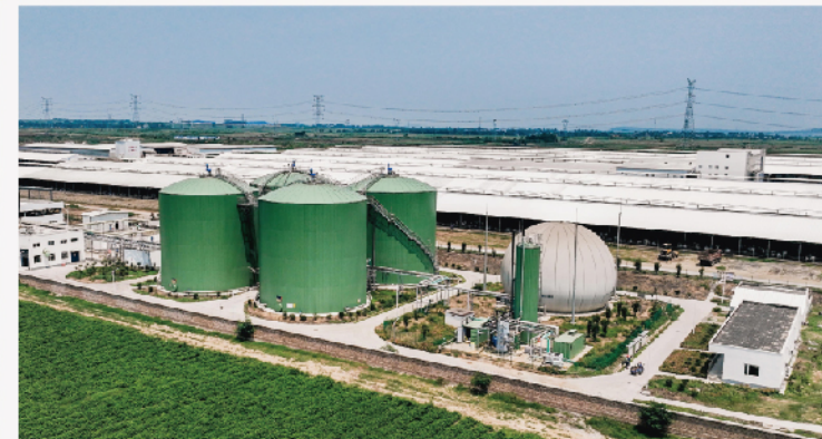
Processing capacity: cow dung 1,000t/d
