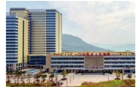
Yunyang County People's Hospital
